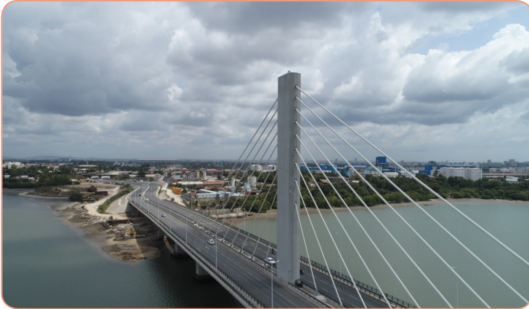
Figure 4.4: Nyerere Bridge in Dar es Salaam, Tanzania
