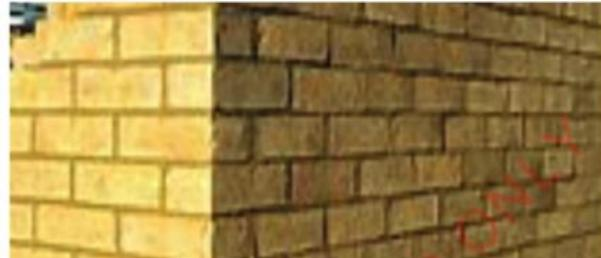
Figure 3.1: Bricks bonded using mortar to form a wall
